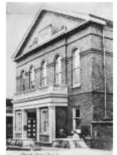
Queen Street Chapel, Sheffield from the website of the Central United Reformed Church, Sheffield.
